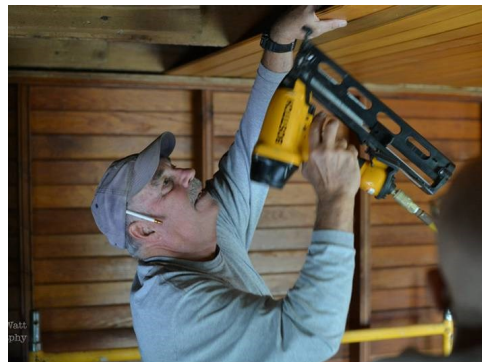
Arvon Byle reinstalls ceiling board in parlor
