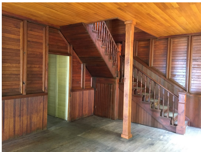
Original wood walls were cleaned, stained, and touched up, restoring the grandeur and beauty of the interior
