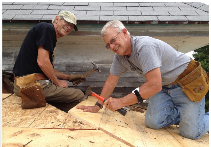
Margo and Libby, (left) cut rough sawn sheathing, while Fred and Doug (above) install it to match the historic material
