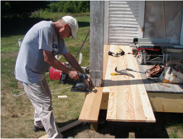
Phil Bergman replaces deteriorated flooring on the porch
