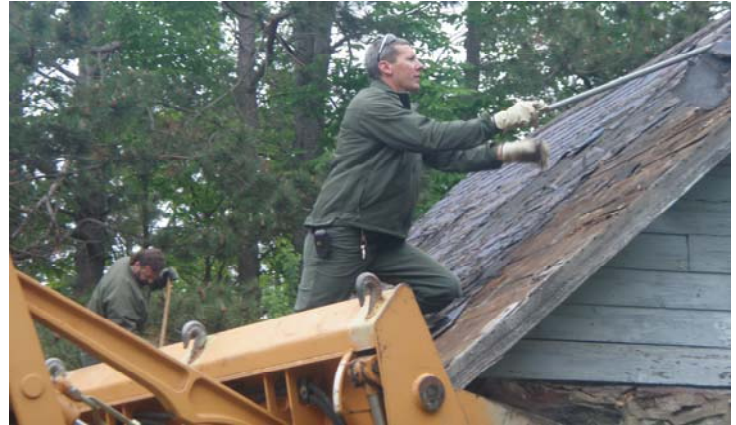
Scott Bigley and Lew King from the Park strip shingles off the stone barn roof at the Werner/Basch farm in the Port Oneida Rural Historic District.
