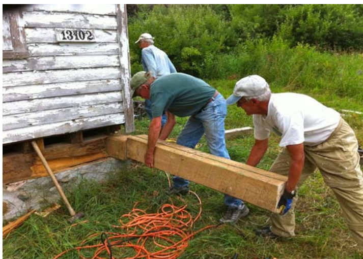
Jack Boss, Doug Detzler and John Sargent replace rotted sills
